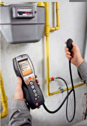
The gas pipe test
